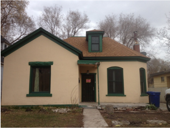
6-Mar-14 14:05 630 E Main St, Salt Lake City UT 12345 Mark Shepard, photographer
