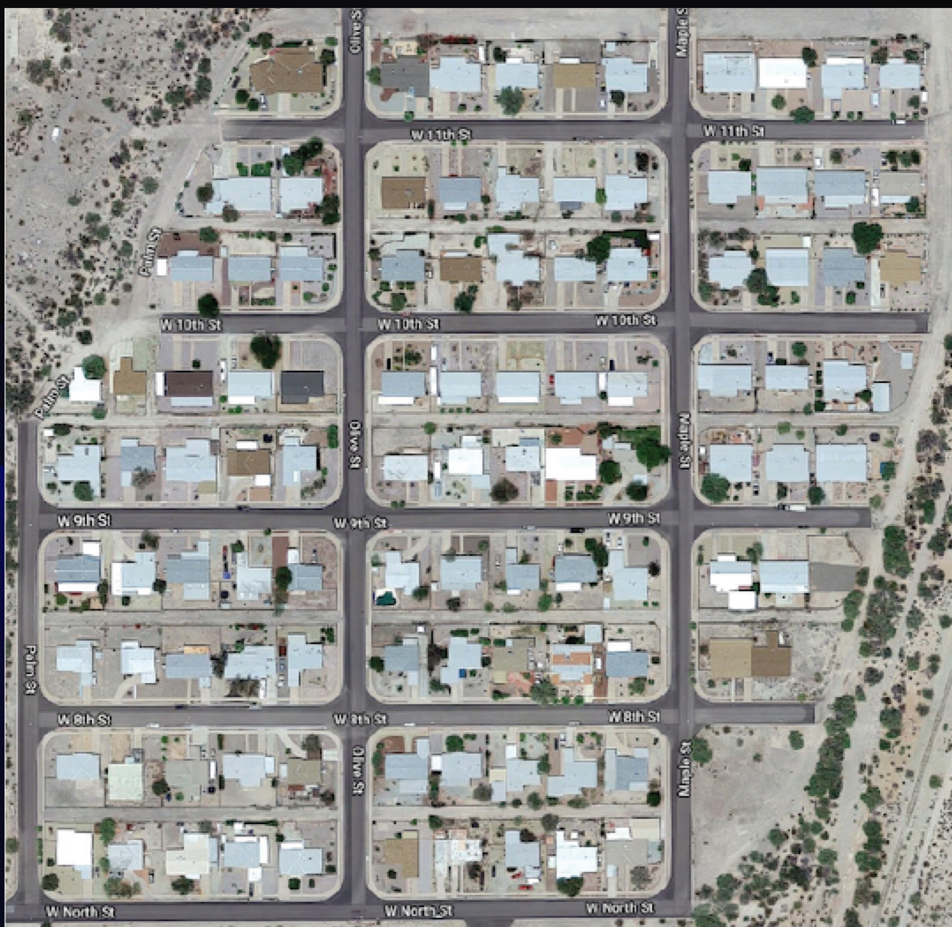
Housing development project from 1972 using AACT system. 115 units constructed in 75 days in Ajo, AZ.
